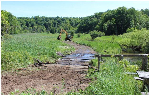
Kanouse Outdoor Restoration laying mats along the stream to access the site for restoration; picture credit John Wyns.
